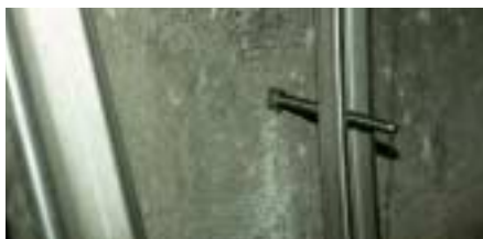
STAINLESS STEEL CLADDING (above) has been used to anchor fibre cement panels to the walls of the tunnel and rock bolts (right), made from round bars of S31603 stainless steel, anchor the stainless steel shapes to the tunnel walls.
