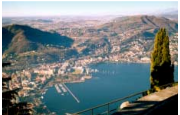
Como, Italy, 30 kilometres north of Milano, where a 33,000-cubic-metre-per-day drinking water plant has been constructed in a cavern inside of Bardello Mountain.
