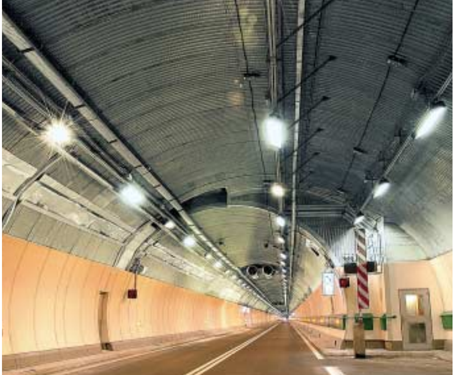
SAFETY IN THE MONT BLANC TUNNEL has been improved significantly through the use of heat- and corrosion-resistant S31603 stainless steel for several key design elements.
