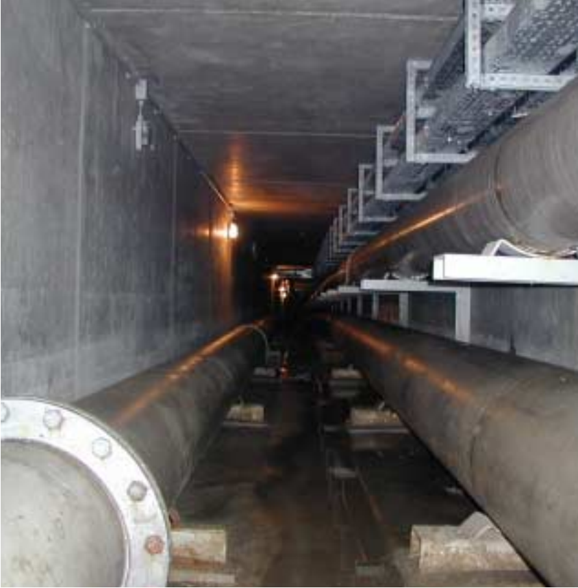
WATER from Lake Como is pumped underground through S30400 stainless steel pipes, 700 millimetres in diameter (above). The use of corrosion-resistant nickel stainless steel should result in lower maintenance. Drinkable water is pumped to a storage tank through stainless steel pipe, 400 millimetres in diameter.
