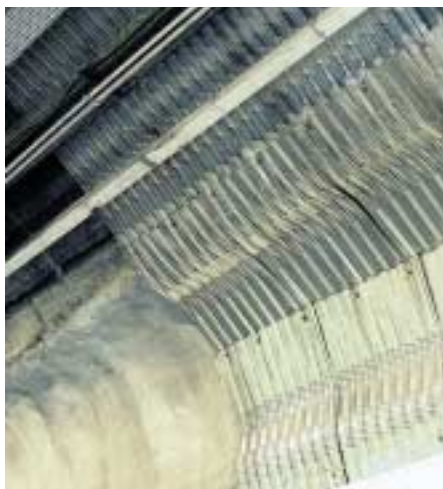
STAINLESS STEEL CLADDING (above) has been used to anchor fibre cement panels to the walls of the tunnel and rock bolts (right), made from round bars of S31603 stainless steel, anchor the stainless steel shapes to the tunnel walls.
