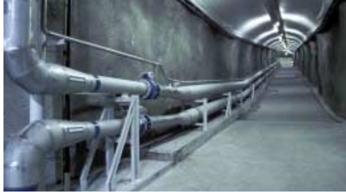
WATER from Lake Como is pumped underground through S30400 stainless steel pipes, 700 millimetres in diameter (above). The use of corrosion-resistant nickel stainless steel should result in lower maintenance. Drinkable water is pumped to a storage tank through stainless steel pipe, 400 millimetres in diameter.
